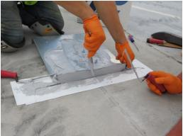
11. Refill the top of the slot with excess epoxy and work out any air bubbles. Strike off excess epoxy to leave a smooth finish.
