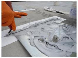
9. With the last of the epoxy left on the mixing board, use pressure filled strokes (think spackling) to cover a cleaned biscuit with epoxy making sure to work the epoxy into the textured surface of the biscuit
