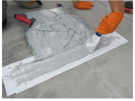
12. Allow the epoxy to set for 5-15 minutes before peeling tape off concrete.
