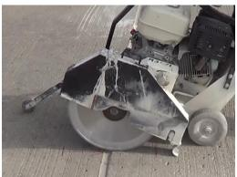
3. With an actual biscuit, make sure the bottom of the cut its level and the proper depth. If dry cut, use an air compressor to clean debris. If wet cut, use a pressure washer to clear debris, then allow 24hr to dry.
